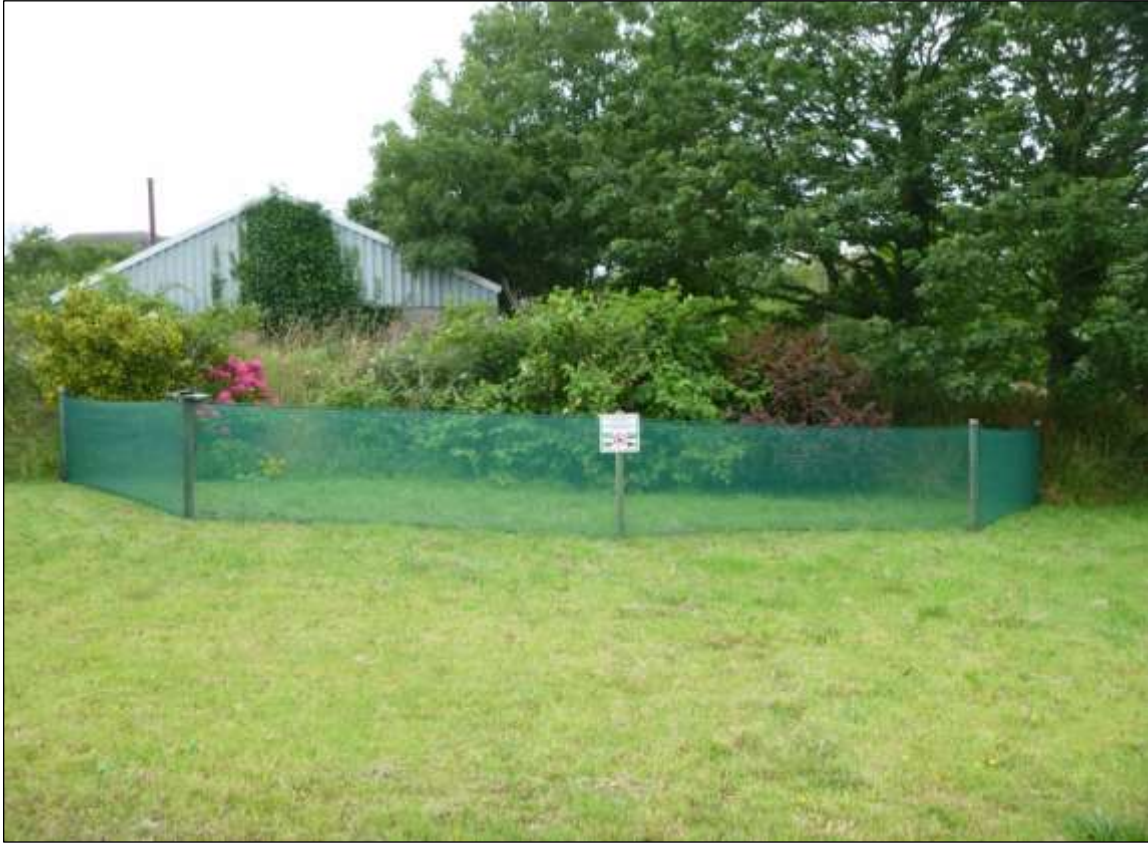
SAMPLE FENCING 1 – POST AND WOVEN MESH FENCING
