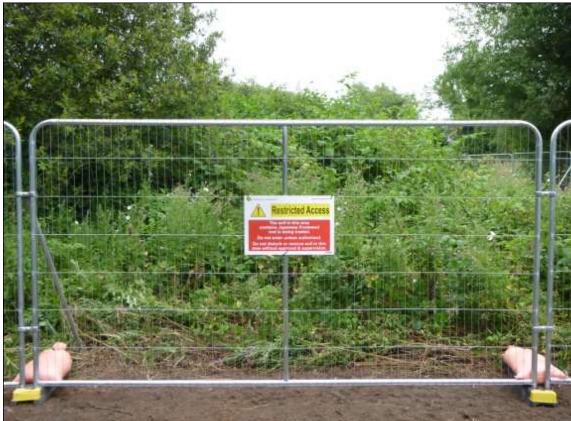
SAMPLE FENCING 2 – HEAVY DUTY HERRAS FENCING
